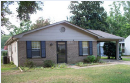
The front of the home before the tornado.
