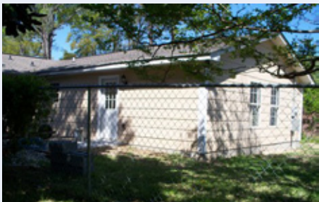
The rear addition is where the safe room was located
